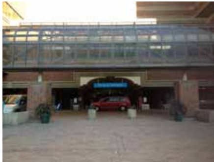
Front (west) entrance of U of A Hospital.
